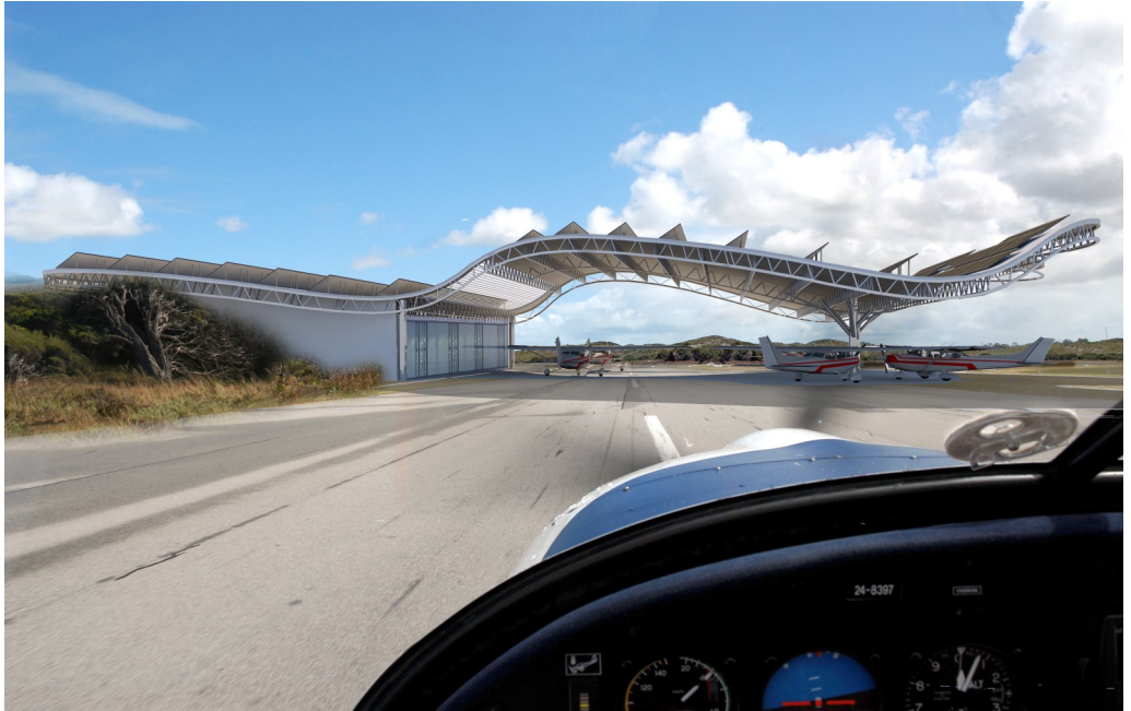
Rottnest SolAirPort – Solar recharge station for the Electro Alpha
